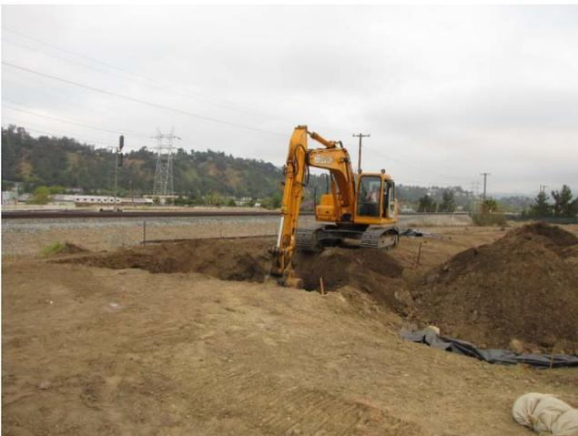
Test Pit/Potholing Excavator
